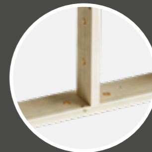
Drill holes in the studs for easier cable threading.
